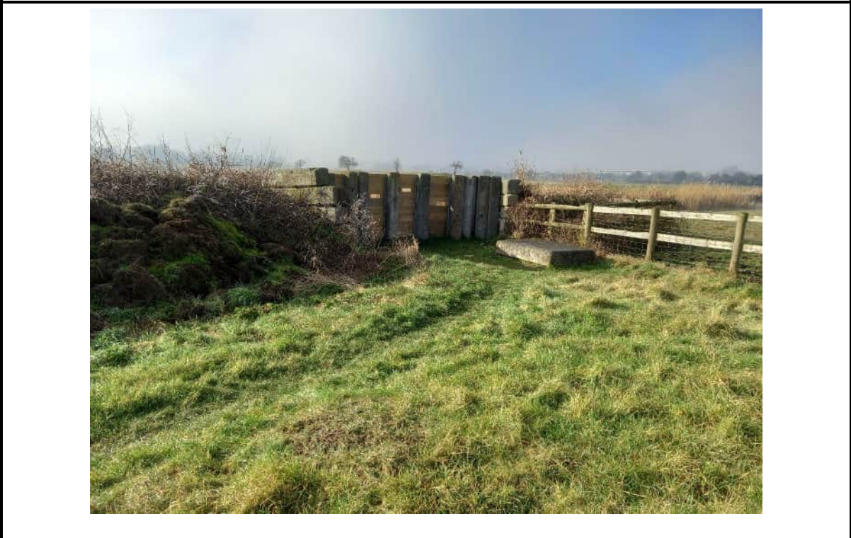
Photo 19: Wood and concrete structure to the west of pond shown in Photo 18.
