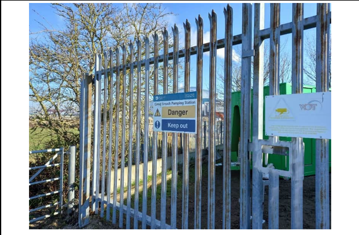
Photo 33: Great Breach pumping station.
