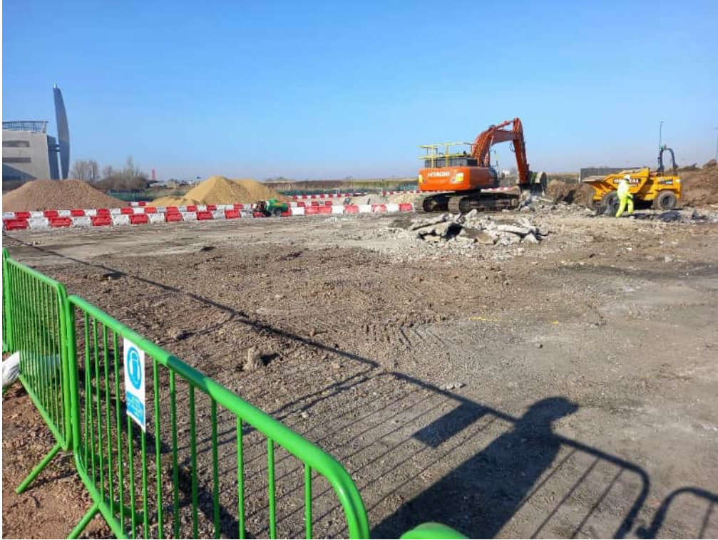
Photo 29: View towards north-west of HZI construction site.
