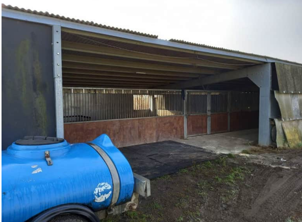
Photo 24: View inside farm infrastructure located in centre of site.
