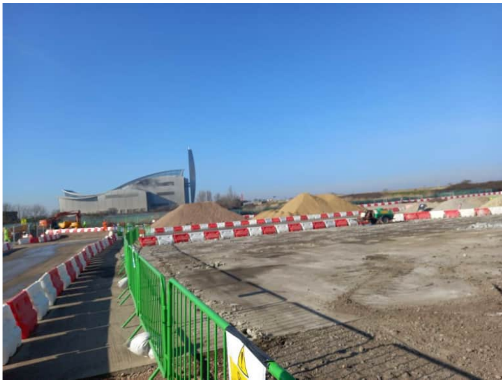
Photo 30: View towards west of HZI construction site.
